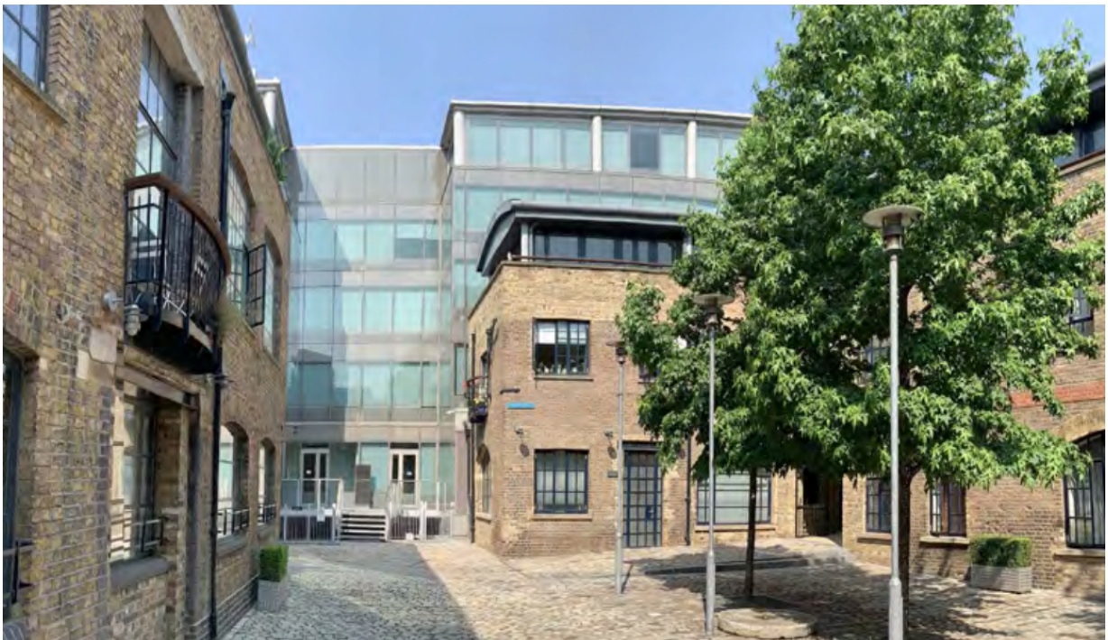
Image 4 – Existing View of Albion Yard
