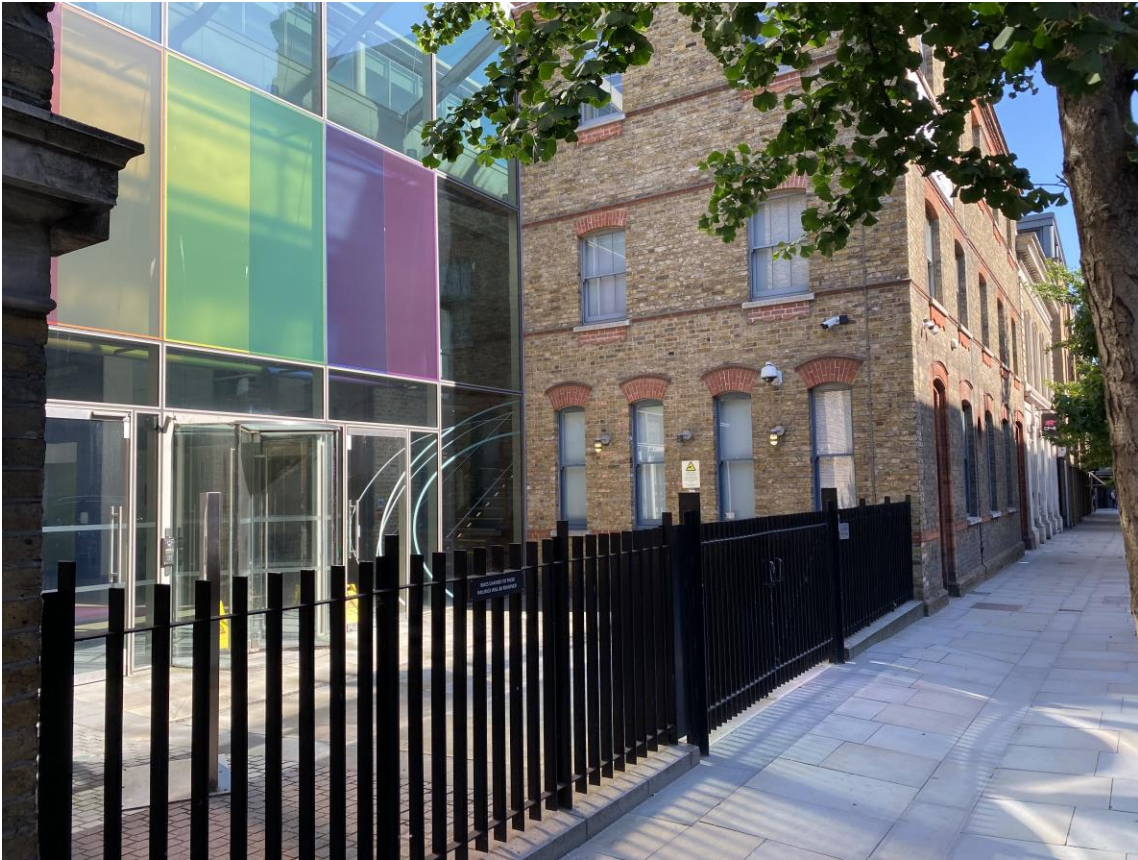
Image 3 - Existing front elevation (looking south)
