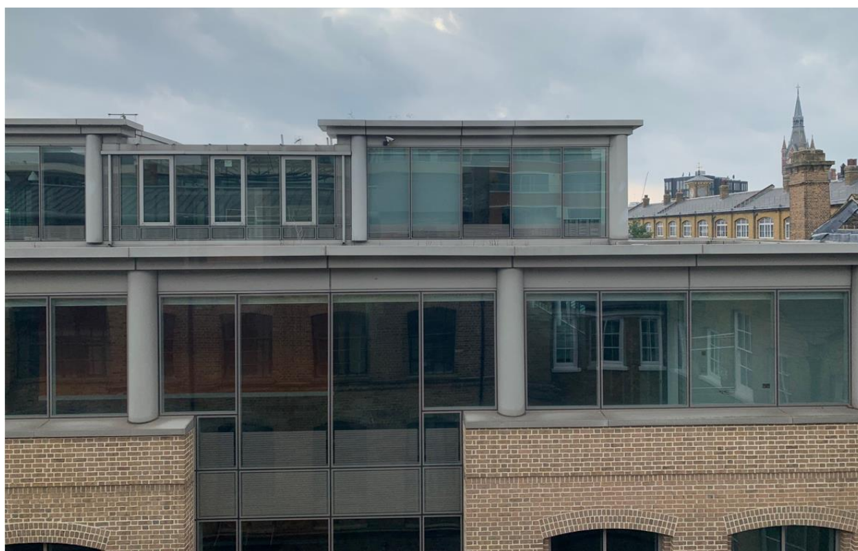
Image 44 – Existing overlooking between The Ironworks and Jahn Court
