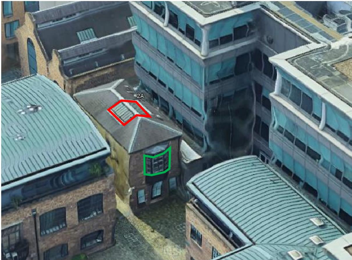
Image 43 – Aerial View of 2a Albion Walk
