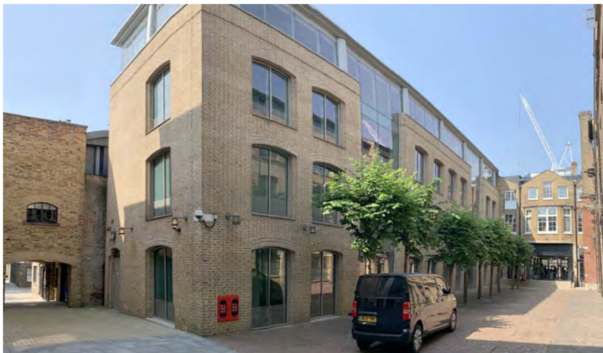
Image 5 – Existing View of Ironworks Yard
